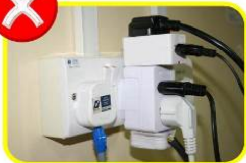
Overloaded sockets - Potential electrical fire hazard
