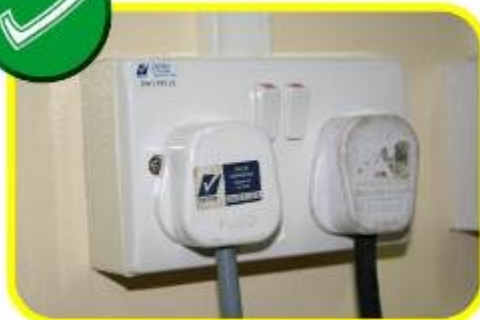
Good practice - Without overloading and causing fire hazard
