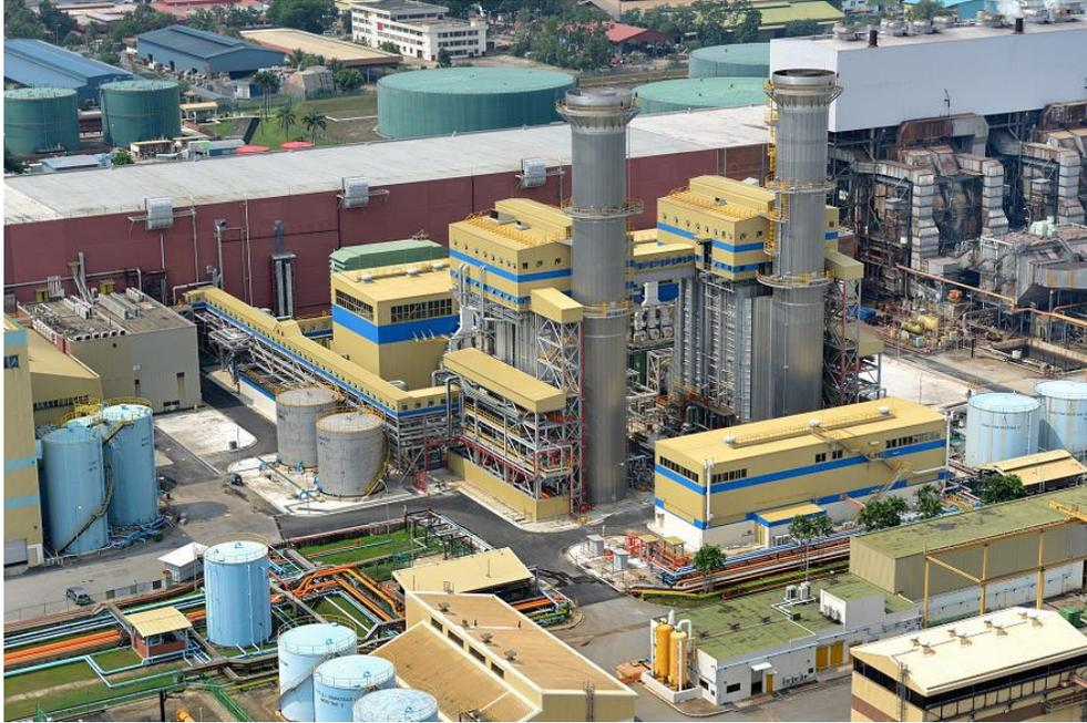
CCP 6 (left) and CCP 7 (right) were constructed on the same site as the former Stage 2 oil-fired plant. CCP 6 and 7 use state-of-the-art gas turbines supplied by Mitsubishi Heavy Industries. The repowering project was completed in the third quarter of 2012.
