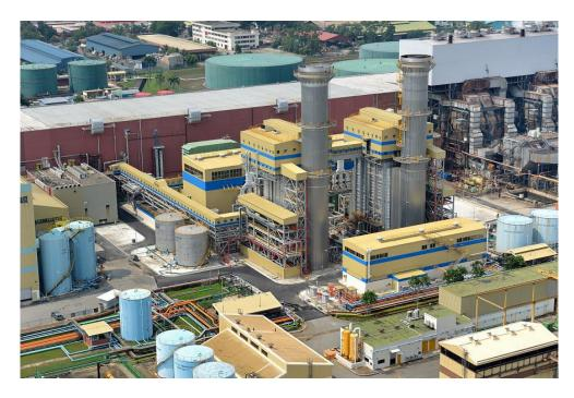
CCP 6 (left) and CCP 7 (right) were constructed on the same site as the former Stage 2 oil-fired plant. CCP 6 and 7 use state-of-the-art gas turbines supplied by Mitsubishi Heavy Industries.
